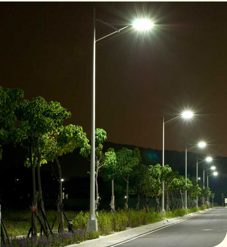
Electrification and street light
