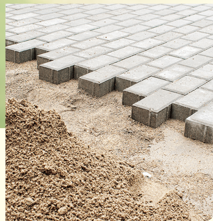
30 feet internal paved road with Drainage system
